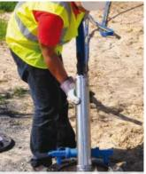
Lower Pump into Bore
